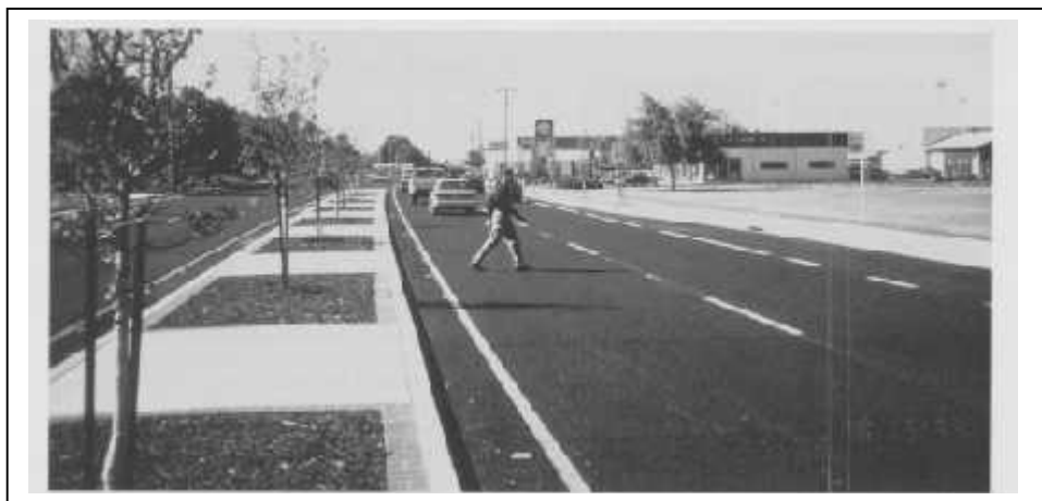
Figure 22. Median allows pedestrian to cross one direction of traffic at a time Source: Oregon Bicycle & Pedestrian Program
