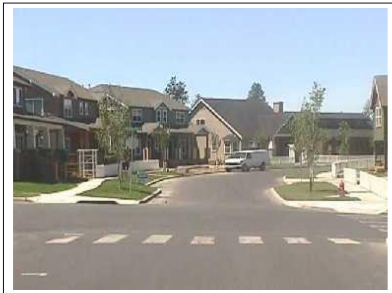
Figure 30. Example of a 20' wide curb extension or "choker" on a 30' wide street
