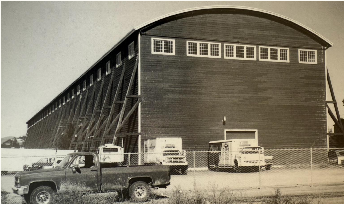
Brooks-Scanlon building converted into a warehouse
