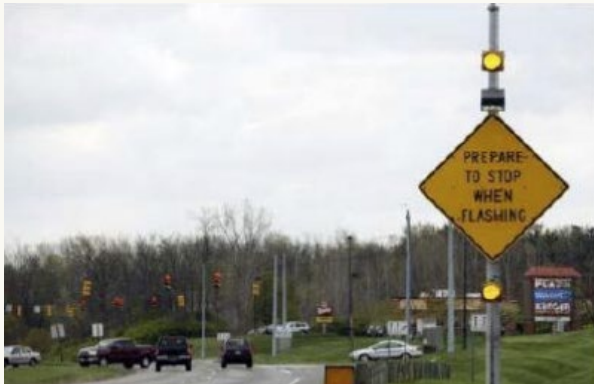
Flashing Beacons Coordinated with Signal
