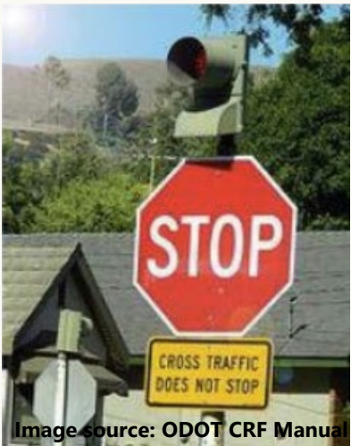
Flashing Beacons on Stop Signs (Potential Crash Reduction = 13%)
