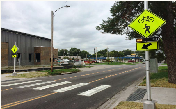
Pedestrian Activated Beacons
