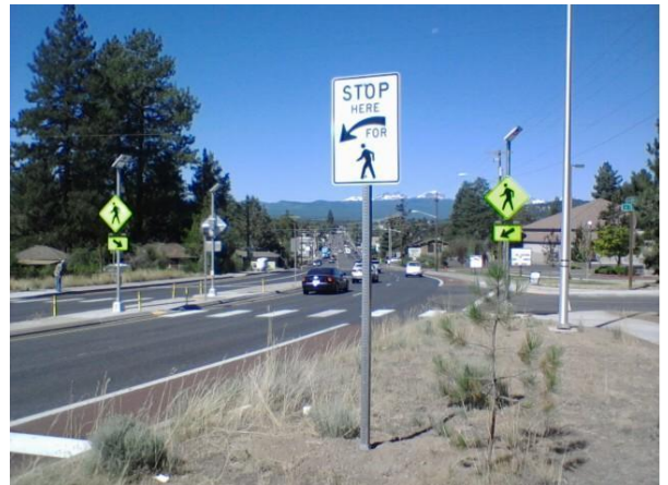
Rectangular Rapid Flashing Beacon (RRFB) at Greenwood Avenue and 12 th Street. As at this crossing, on four-lane arterials it is important to provide a raised median with pedestrian refuges.
