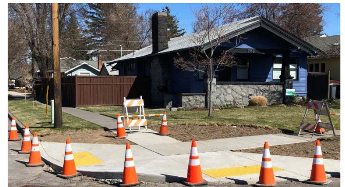
Figure 3 NE Corner Delaware/Sisemore (new ramps spring 2020)
