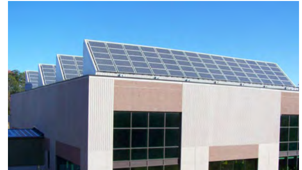
Photovoltaic panels integrated into a building's industrial architectural form.
