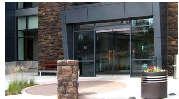
Natural, local materials highlight a main entrance.
