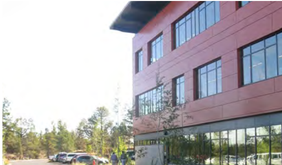
A clear pattern of windows establishes the facade's set of proportions.
