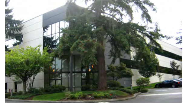
Mature tree is saved, even close to building.
