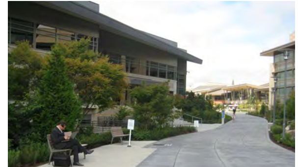
Walkways link different buildings.
