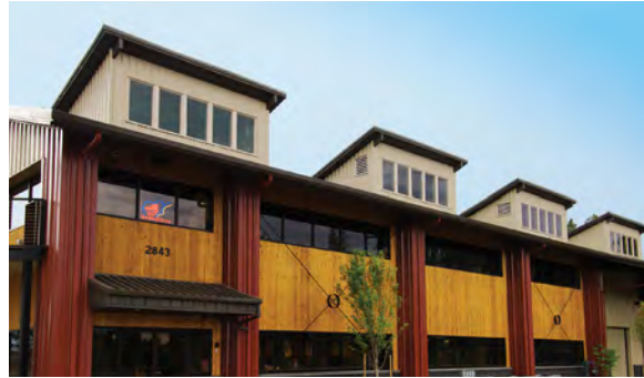
Light monitors create distinctive roof forms
