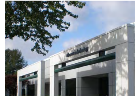
Simple framing elements can create shadow lines that enliven an otherwise plain facade.
