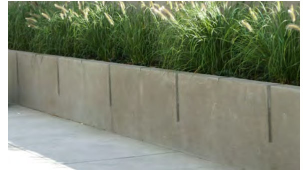
Cast-in-place concrete retaining wall with integrated planters
