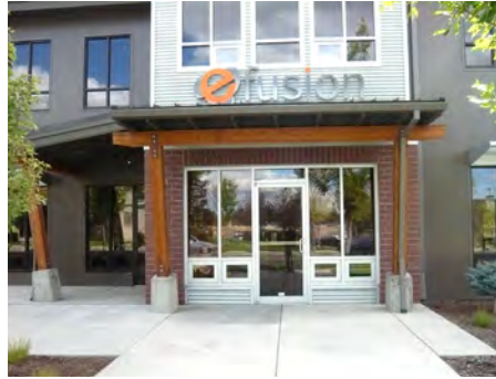
This otherwise simple building incorporates window overhangs, a portico style entry, and larger windows at the base.
