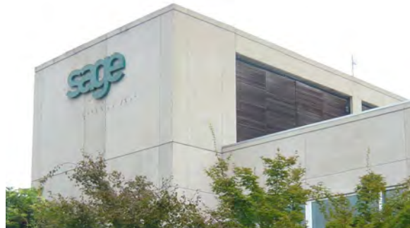
Mechanical space as extension of architecture.
