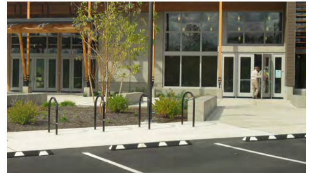
Bike racks close to building entry
