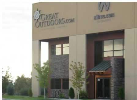
Details at the entrance to large warehouse building.
