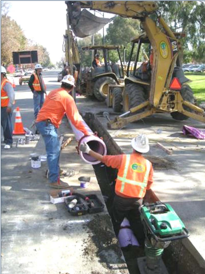
Cut and Cover Trenching
