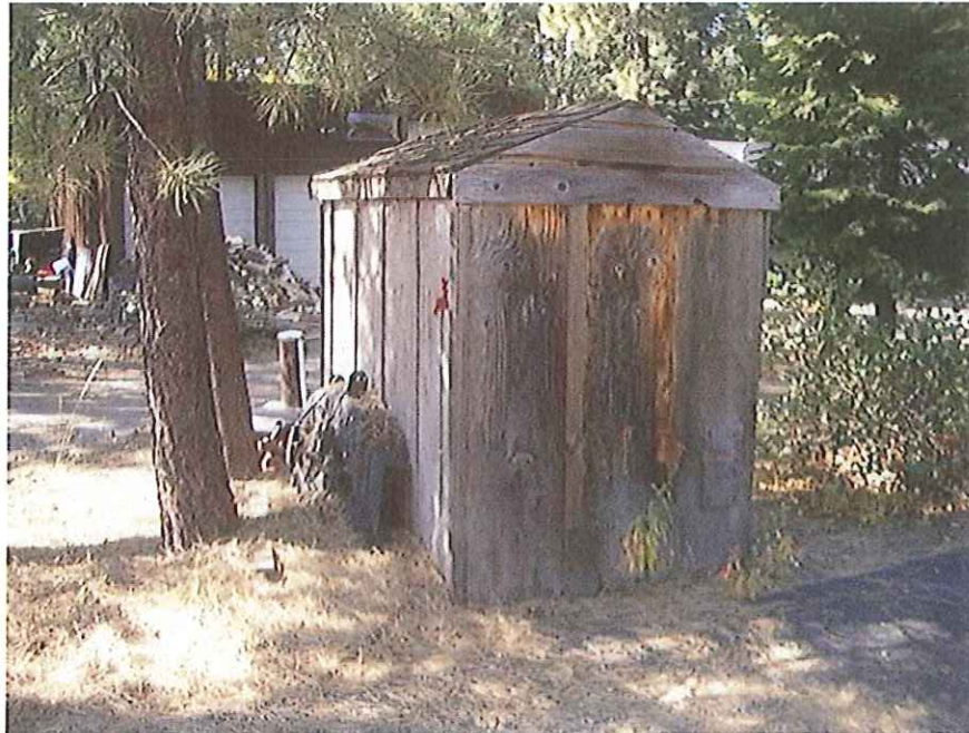
Figure 10. Well house directly above 1926 pipeline; another well can be seen in background that is less than 1 foot from the pipeline
