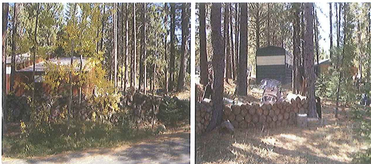
Figure 8. Pipeline route is under right edge of building (left); pipeline route (blue stake) directly under large RV shelter (right)
