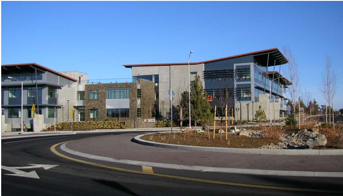
Les Schwab Headquarters at Juniper Ridge
