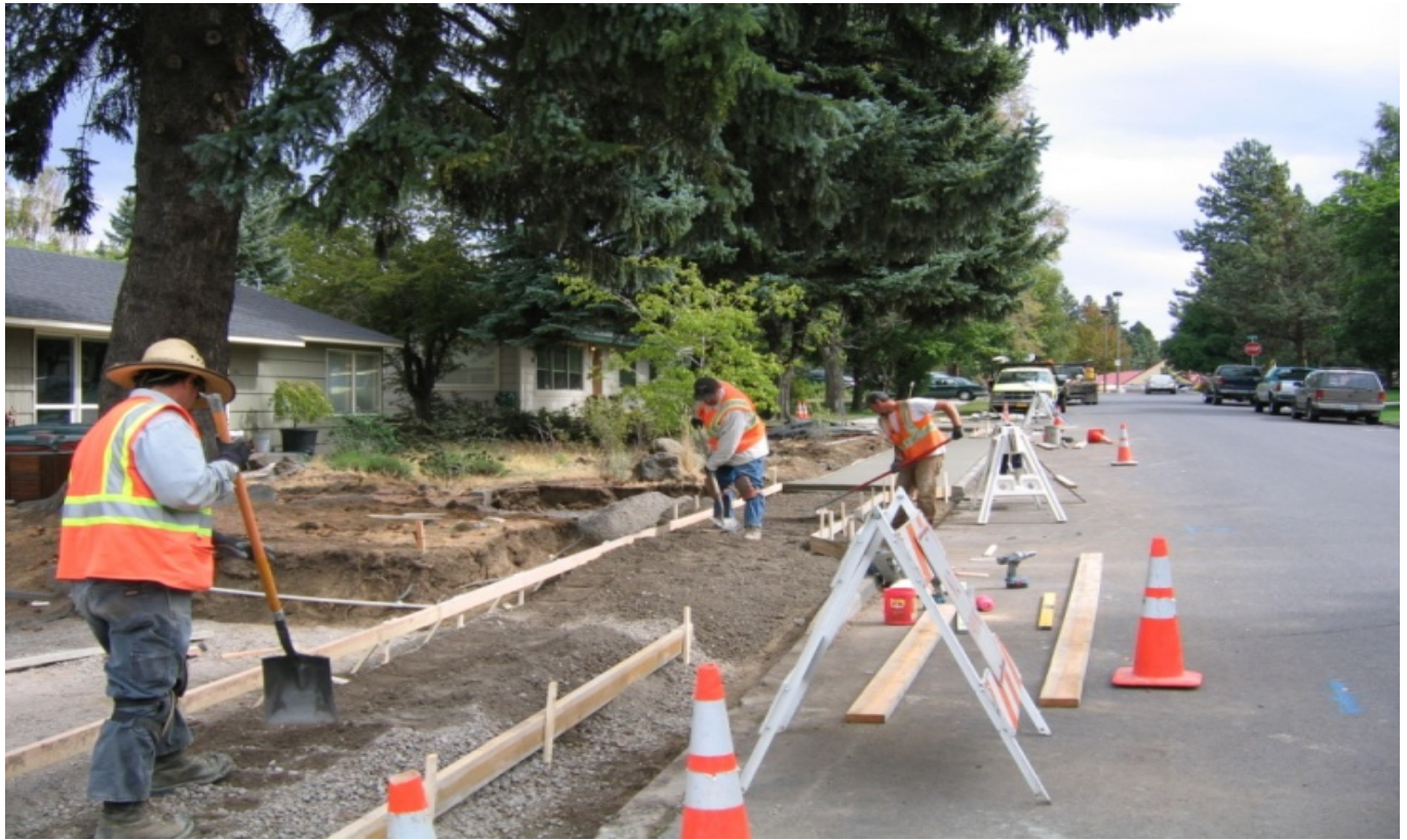
New Sidewalk Construction
