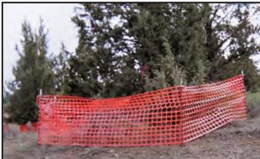
Source: City of Bend
