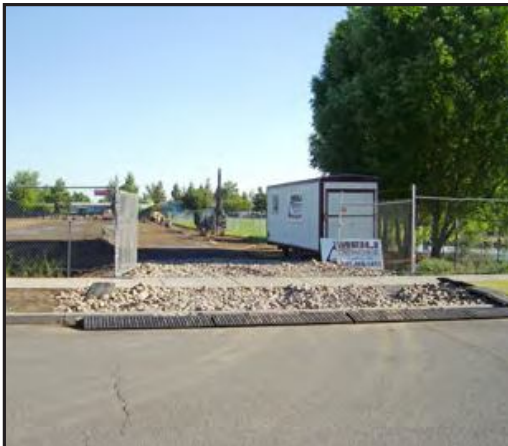
Source: City of Bend
