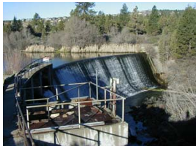
Figure 3. North Canal Dam at approximately 30 cfs
