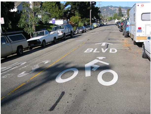
Figure 5.7 Large pavement markings
