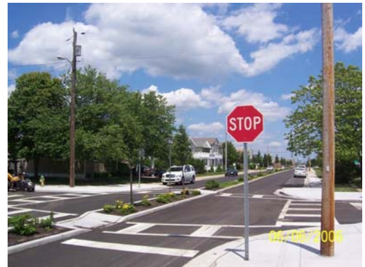
Figure 5.11 Landscape medians restrict motorist movements
