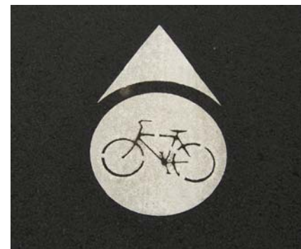
Figure 5.18 Pavement markings with arrows are used to guide cyclist through turns along the bikeway
