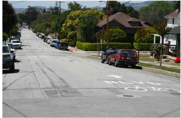
Figure 5.1 Pavement markings and signage identify the street as a bicycle boulevard.
