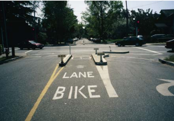
Figure 5.6 Bicycle activated signal
