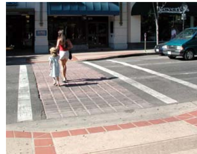
Patterned Crosswalk at Mid-Block Crosswalk
