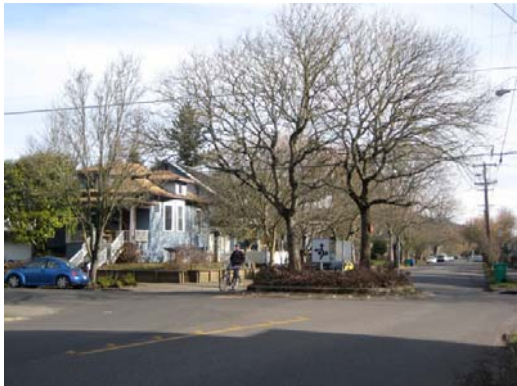
Figure 5.14 Landscaped traffic circles eliminate the need for stop signs at several intersections
