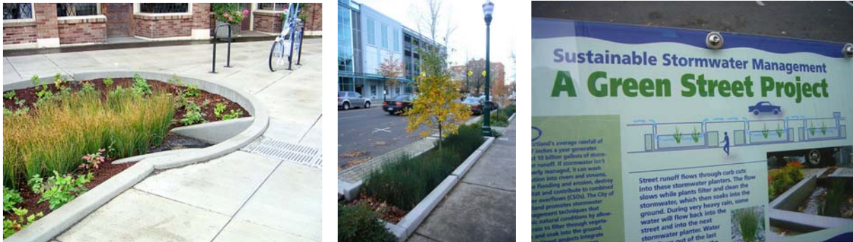
Figure 3.4 A Green Streets project in Portland, Oregon sustainably manages stormwater, slows traffic, and creates a welcoming and pleasant environment for bicyclists and pedestrians
