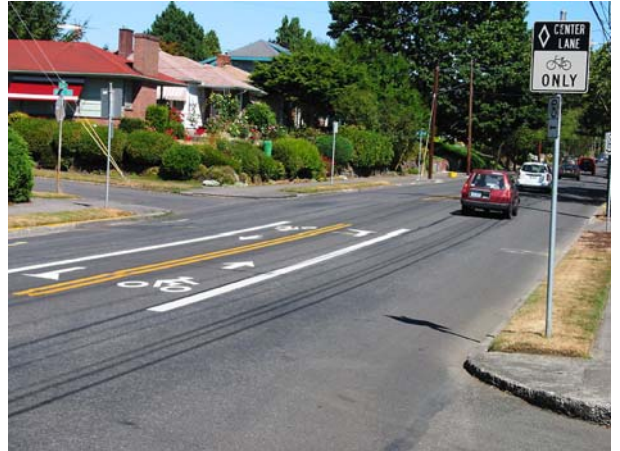
Two Way Center Left Turn - Portland, Oregon
