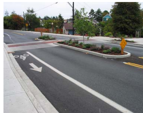
Crosswalk and Median Refuge
