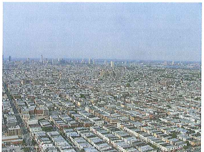
South East Philadelphia, PA. © 2004 Philadelphia Water Department
