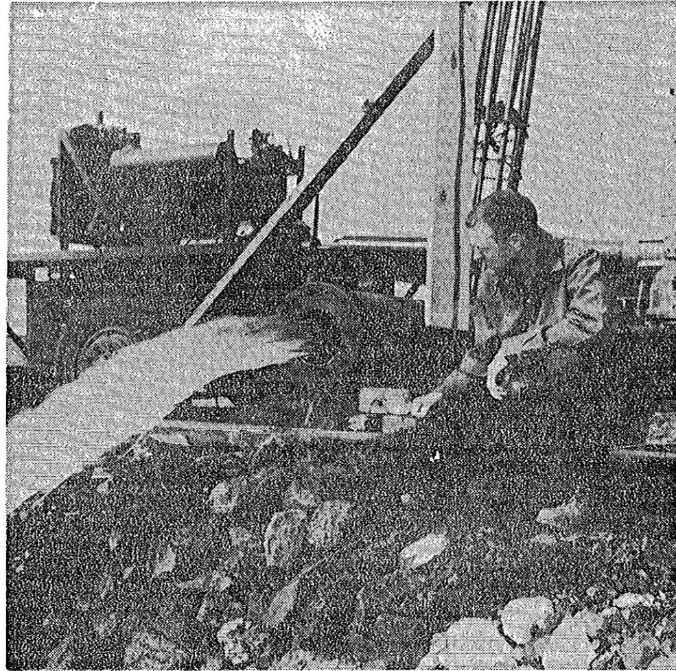
OUT OF THE DEPTHS — Water pumped from a 900-foot well is pictured flowing from a big pipe in a test now in progress across the Deschutes from the Brooks-Scanlon, Inc. plant. Larry Brown of the Brooks-Scanlon staff is shown watching the 1300-gallon per minute flow. The deep well was drilled by Brooks-Scanlon in studies preliminary to the possible establishment of a pulp operation in the area. Engineers said the deep well tests are most encouraging.
