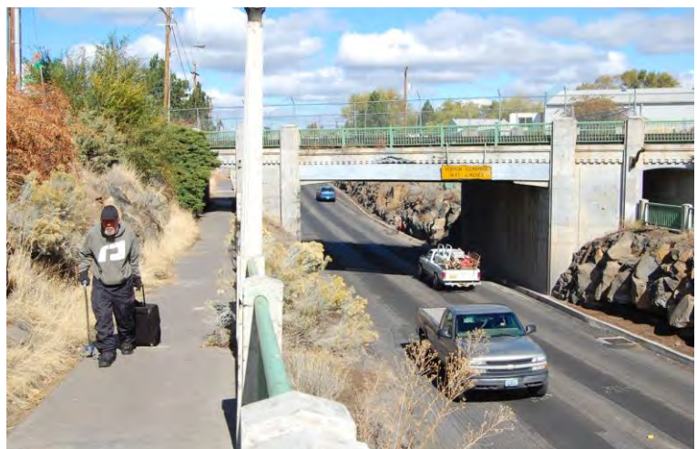
VIEW LOOKING SOUTH ON 3 RD STREET UNDERNEATH RAILROAD
