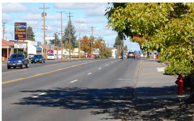
This photo of 3 rd Street at Franklin (looking north) illustrates the need for streetscape improvements, access management (fewer driveways), wider sidewalks, and more frequent designated pedestrian crossings.
