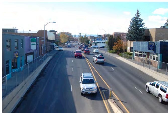
Greenwood, from overpass, looking east Source: SERA
