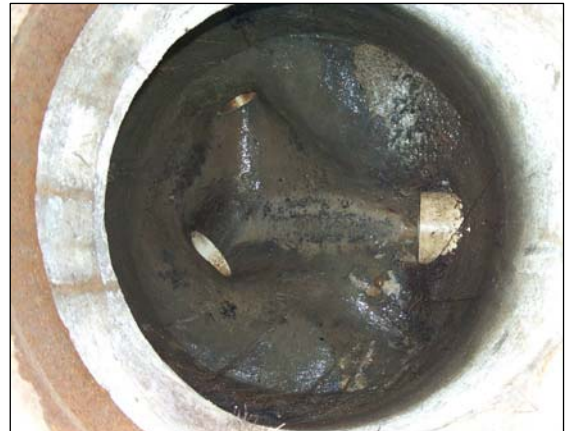
Figure 11: Awbrey Glen PS Discharge Manhole
