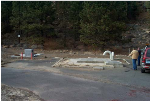
Figure 10: Awbrey Glen Pump Station
