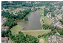
Lake Barton (PL566 Facility)
