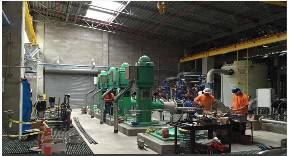
Project Engineer: Heidi Lansdowne | hlansdowne@bendoregon.gov
