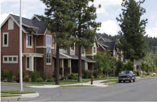
Top: Mixed-use development with office, retail and residential Bottom: Attached townhomes oriented towards street front
