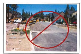
Sediment is not allowed to come off any construction site, whether or not your site is required to have an erosion and sediment control plan or a grading and drainage permit. For additional information, review the Central Oregon Stormwater Manual, Chapter 9 and the "ACWA Construction Site Stormwater Guide" (see Other Resources, below).
