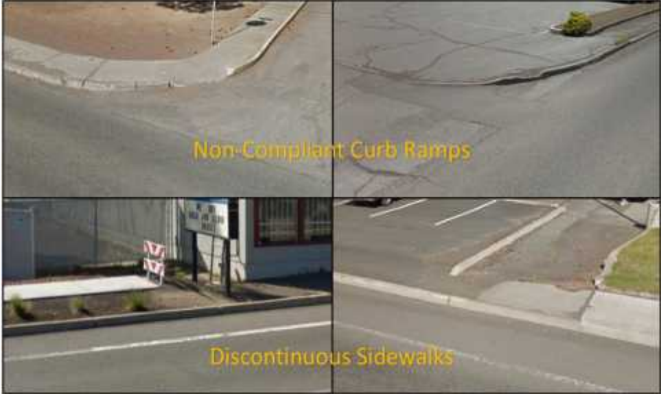
MPO staff assisted the City of Bend to develop a grant application and secure funding to construct sidewalks, curb ramps and transit stops along 3 rd Street, a former state highway. Construction of the improvements will occur in summer 2016.
