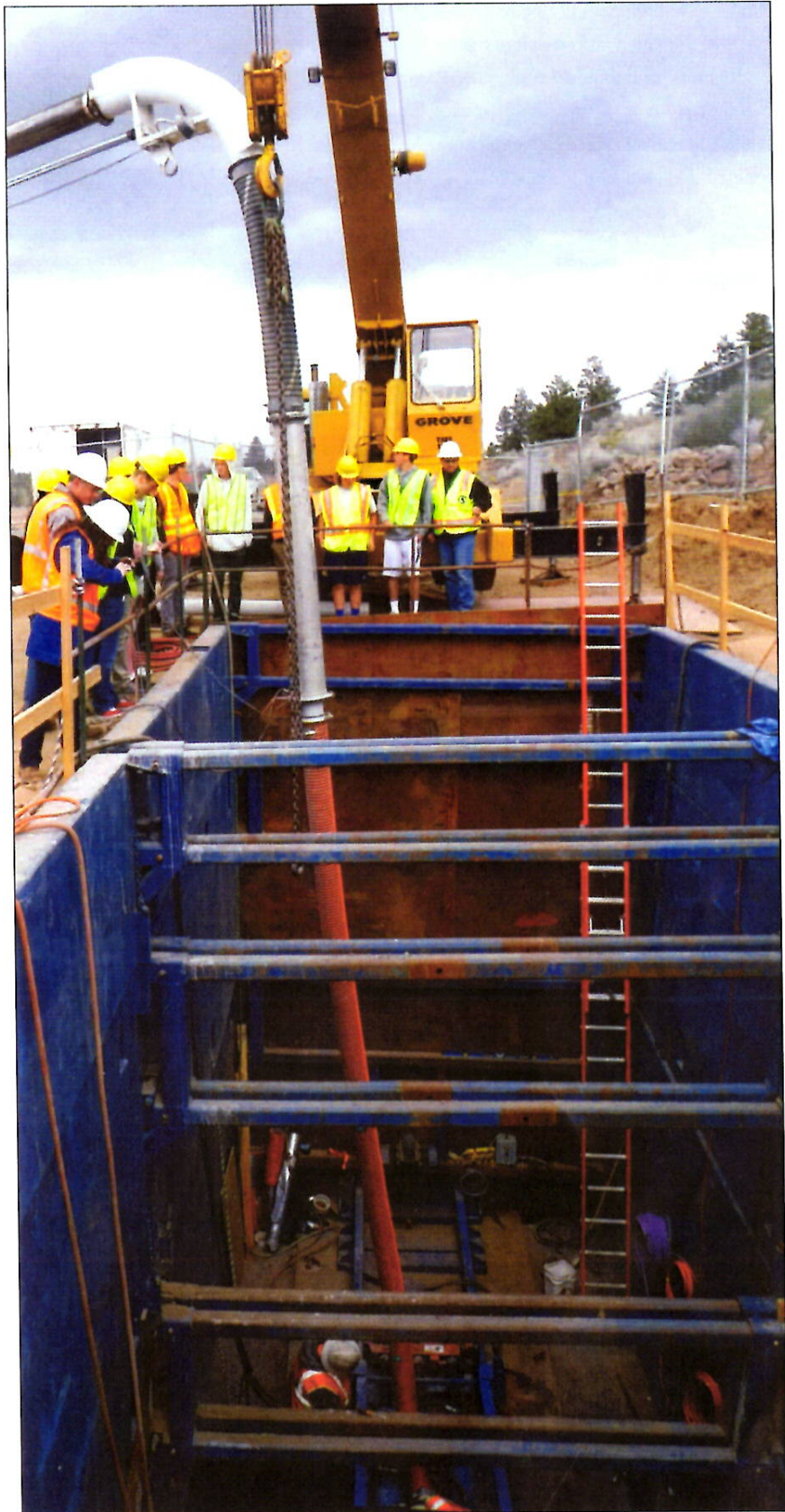
Spoils are removed from behind the SBU-RC cutterhead directly to the surface using a vacuum truck.
