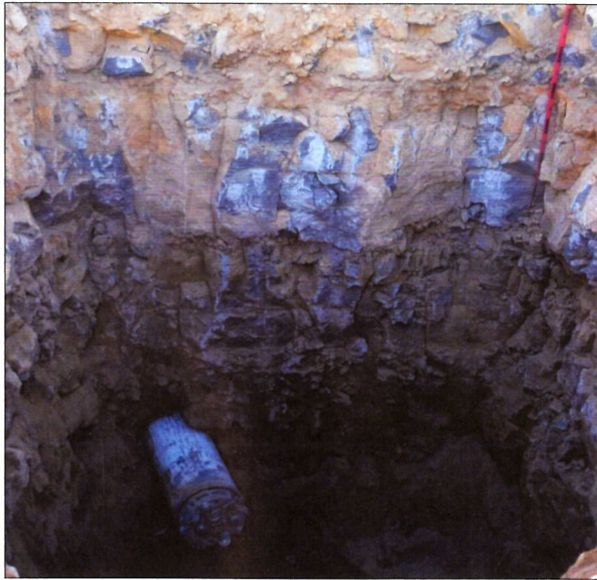
The Robbins SBU-RC broke through two weeks ahead of schedule on May 5, 2015. The blocky basalt subsurface conditions are seen here at the exit pit.
