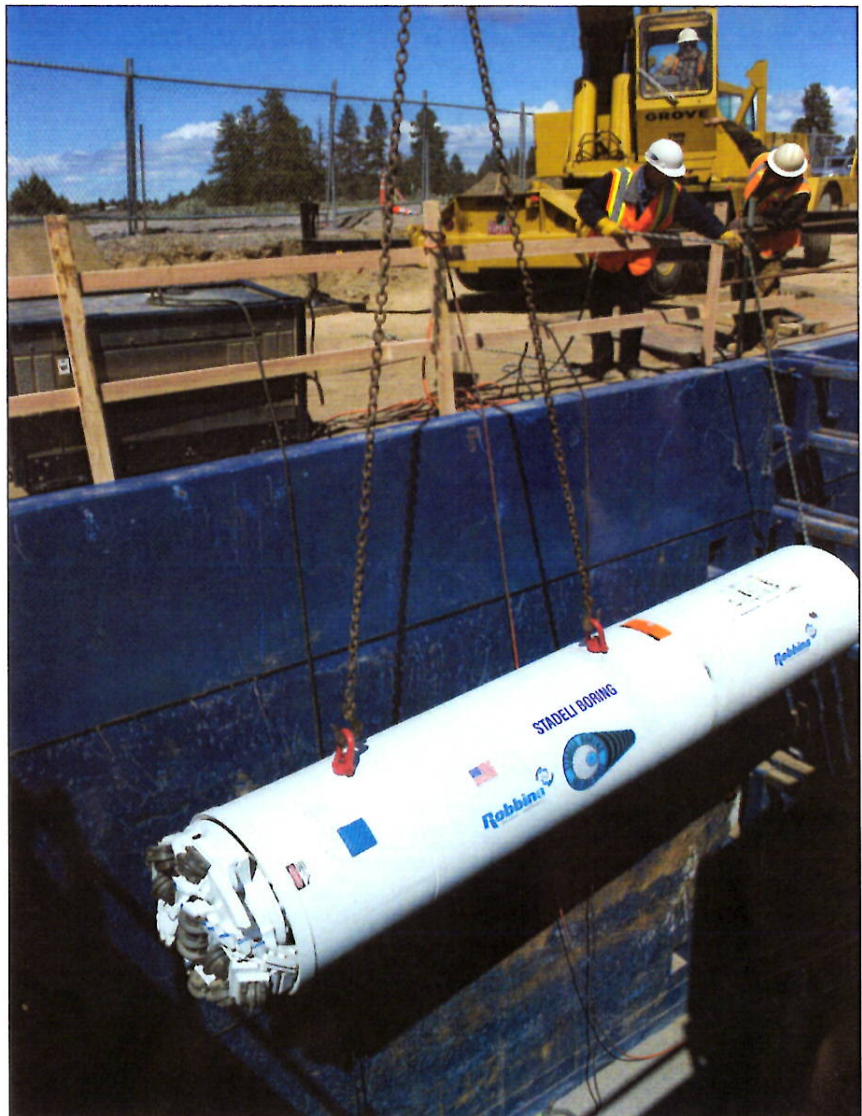
The Robbins 36-inch-diameter SBU-RC was launched at a jobsite in Bend, Oregon, for contractor Stadel Boring & Tunneling in April 2015.
