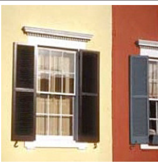
FIGURE 18.1 Delicate muntins and multi-pane sash on early 19th century row houses. Photo Courtesy National Park Service.
