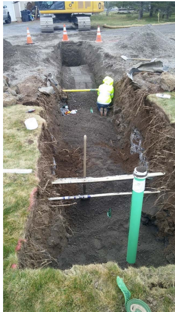
Sewer pipeline stub out for residential connection.
