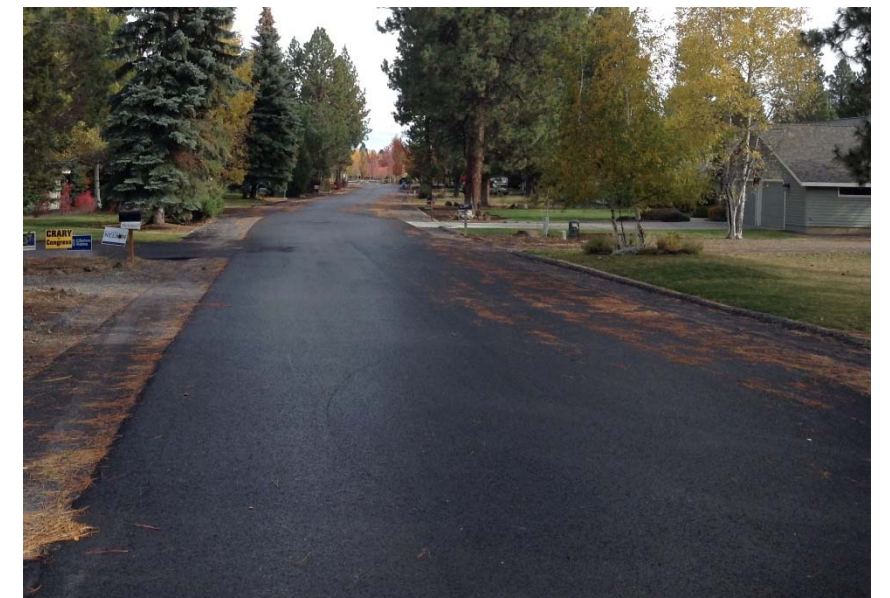
Roadway post construction pavement.
