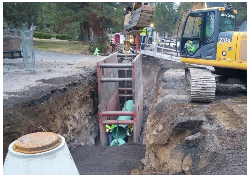
Sewer gravity pipeline construction.
