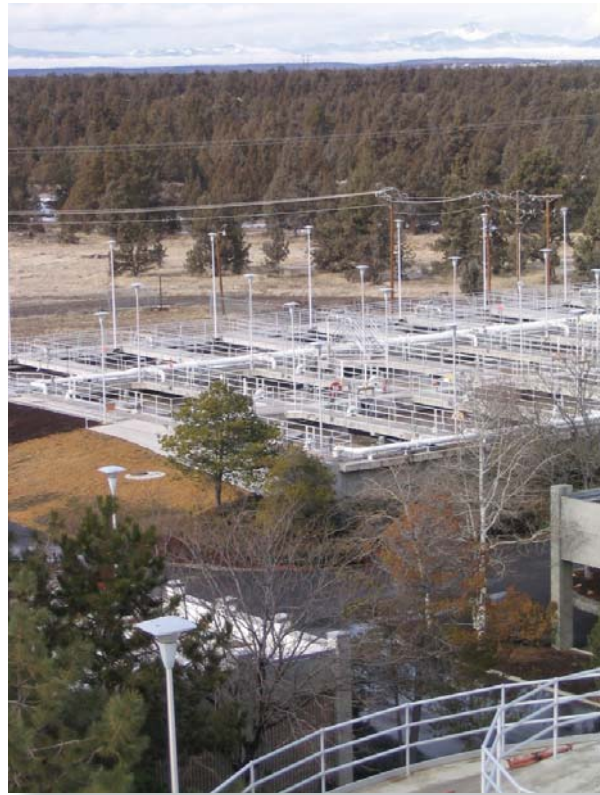
Existing aeration basin capacity will be maximized by adding upstream "filtrate reaeration" basins.
