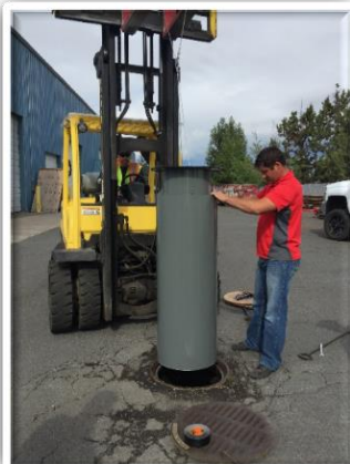
Installing open grate UIC retrofit at Boyd Acres corporation yard as an installation demonstration.
