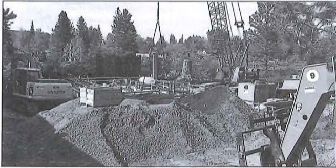
Colorado Lift Station construction
