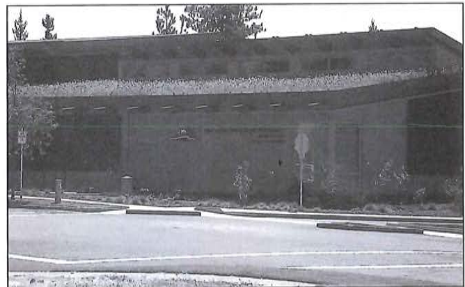
Bend Parks and Recreation admin building green roof
