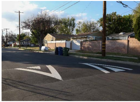
Example of speed hump
