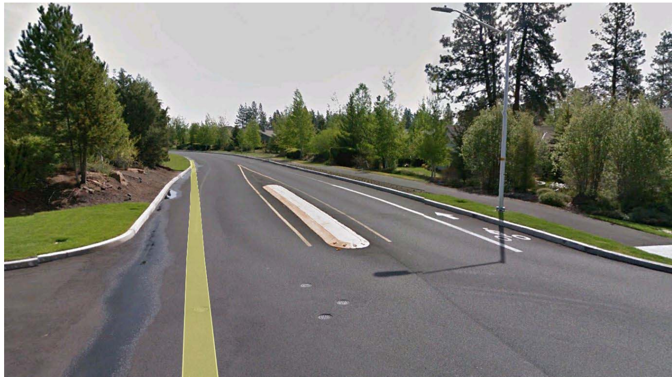
Median Safety Island Example
