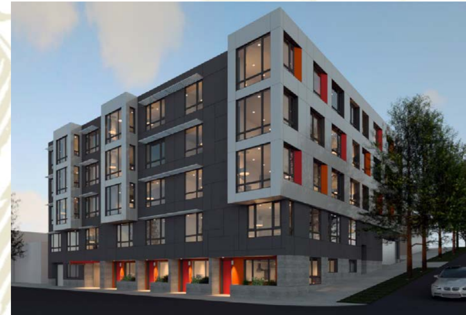
4-over-1 Example: 28 th and Belmont GreenLight Development, Portland
