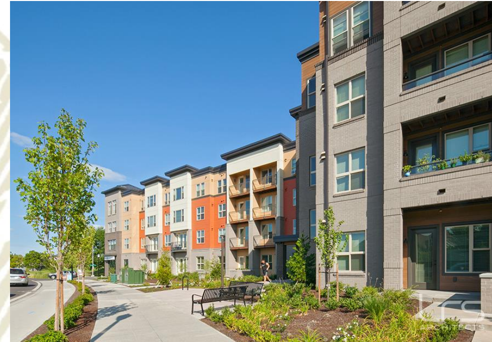
4 Story Wood-frame Example: Nexus, Simpson Housing, Orenco Station, Hillsboro
