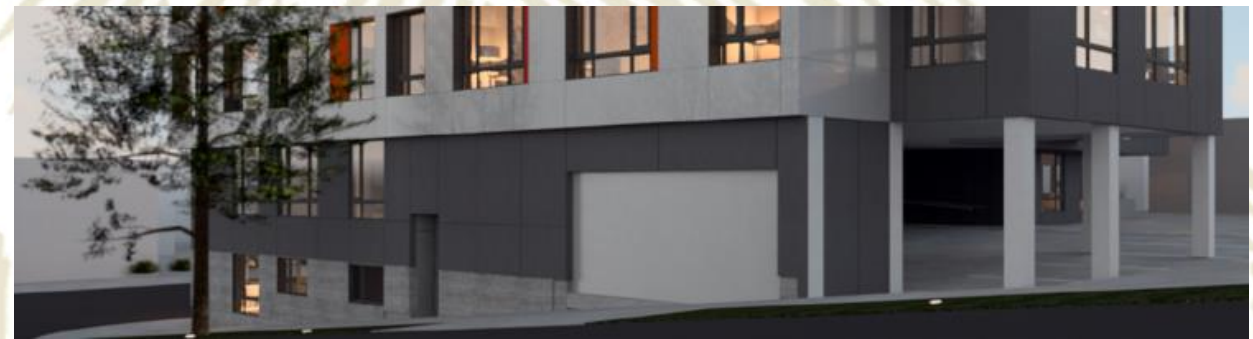
4-over-1 Example: 28 th and Belmont GreenLight Development, Portland
