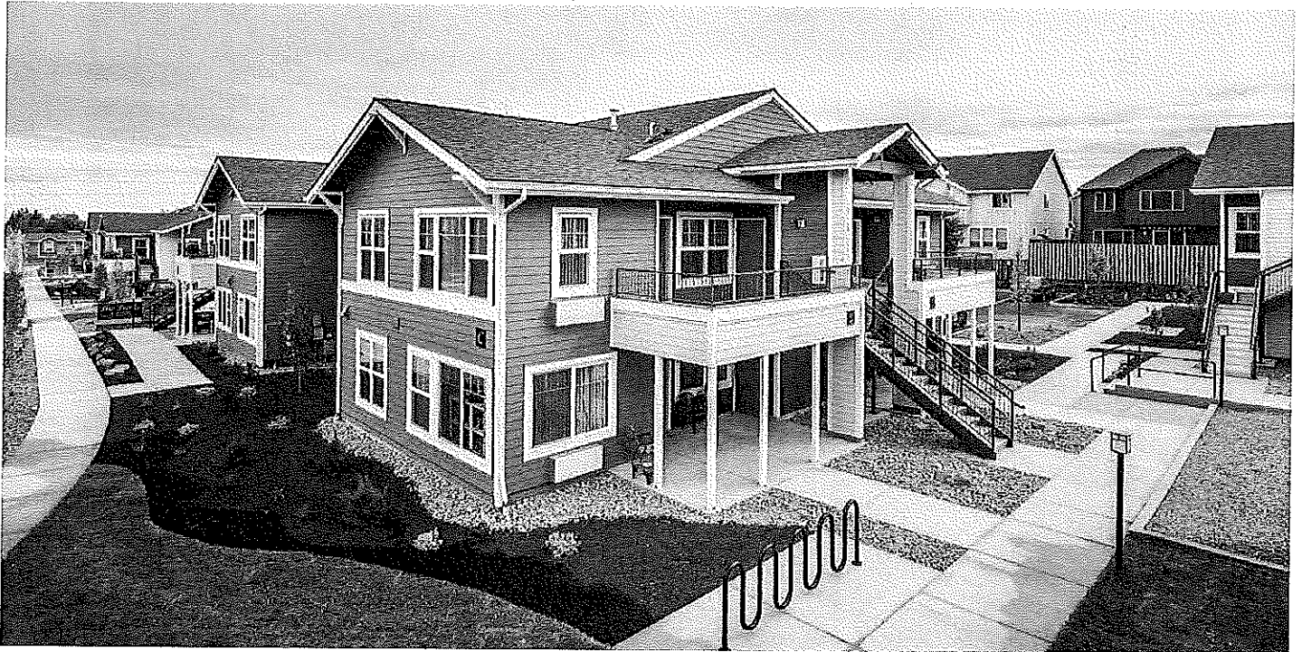
Example of a 2-story affordable housing unit adjacent to RM single family housing within a mile of the proposed site.
