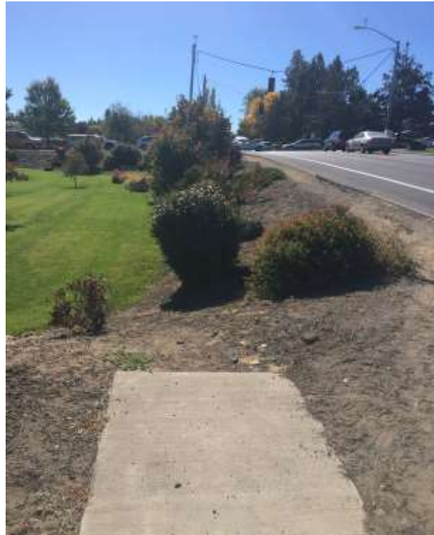
Figure 10. Purcell Boulevard missing sidewalks (facing south toward Neff Road)
