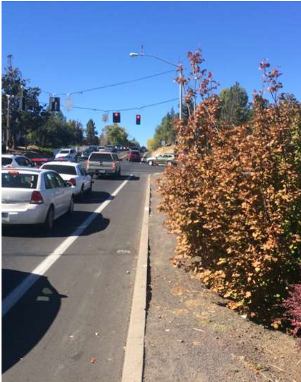
Figure 9. Neff Road missing sidewalks (facing west toward Purcell Blvd)
