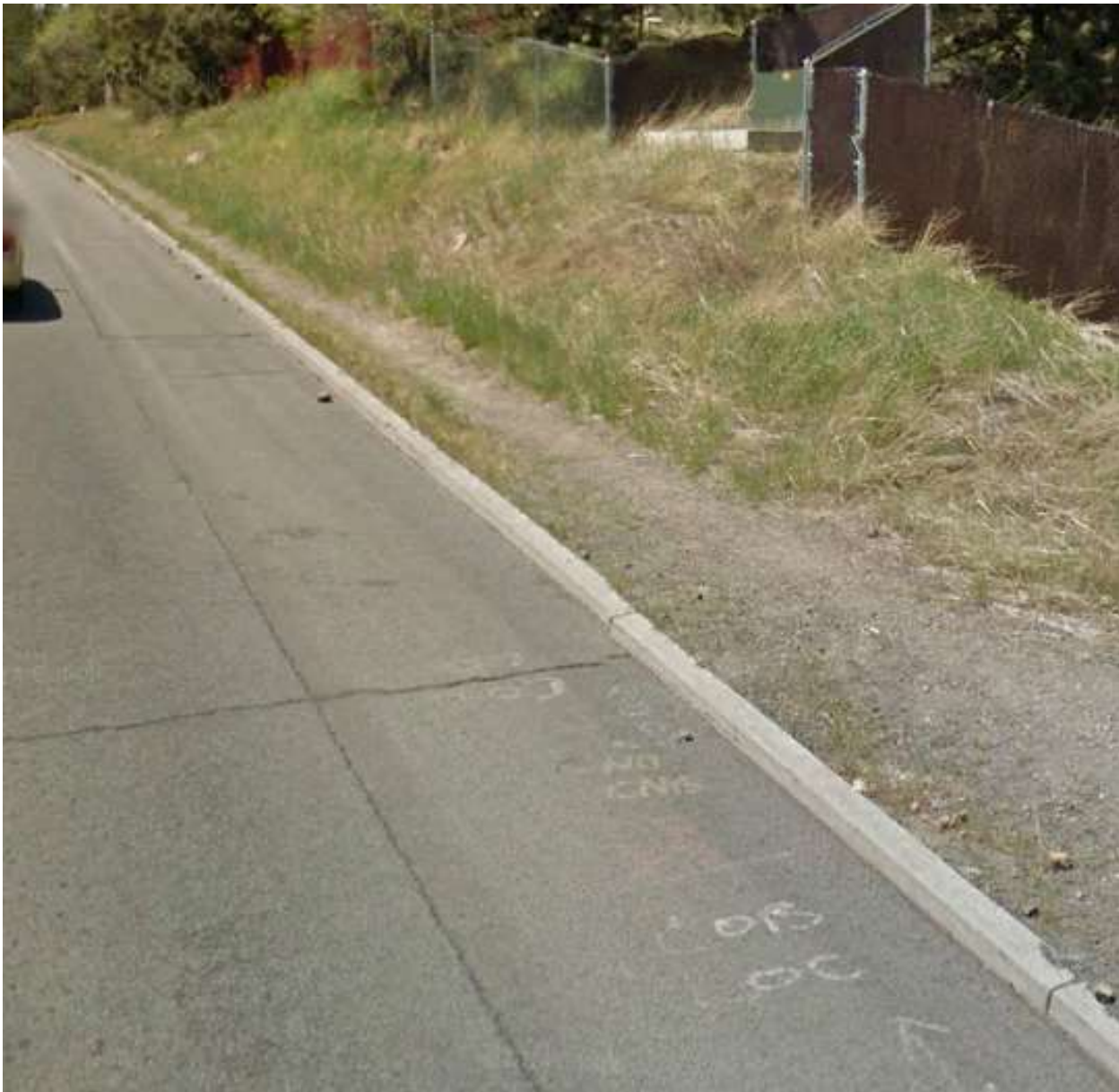
Figure 11. Missing sidewalks on the north side of Neff Road.
