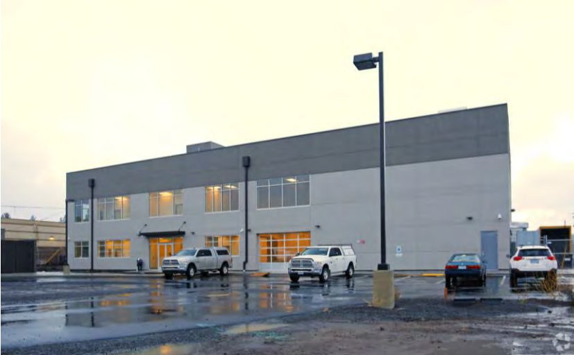
Building Type: Flex Year Built: 2016 Tenant: Data Center Size: 13,500 SF
