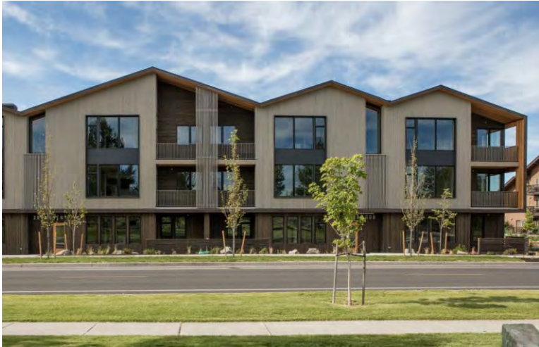
Building Type: Market Rate Rental Year Built: 2017 Units: 132
