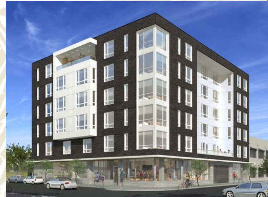
5-over-1 Example: Hoyt 20, GreenLight Development, Portland
