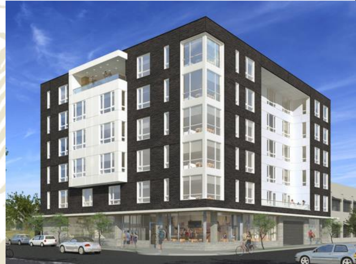
5-over-1 Example: Hoyt 20, GreenLight Development, Portland
