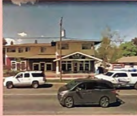
NW Newport Avenue
