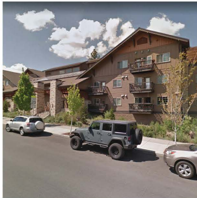
NW Crossing Drive
