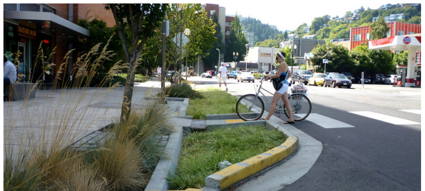
Mid-block crossing, curb extensions, stormwater treatment
