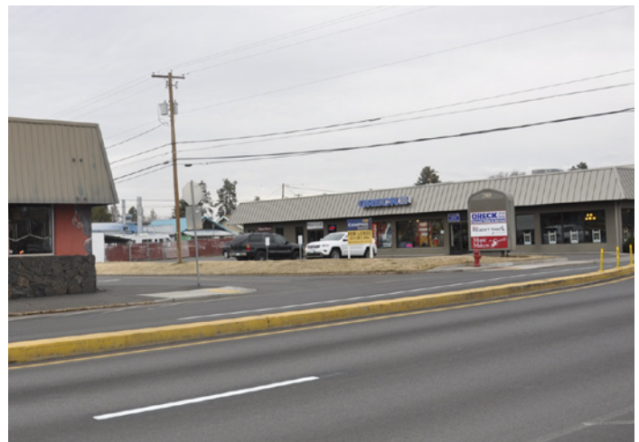
Greenwood high speed traffic and median curb is pedestrian barrier
