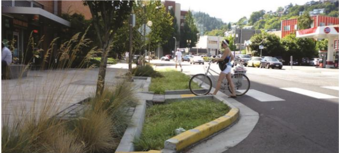
Mid-block crossing, curb extensions, stormwater treatment
