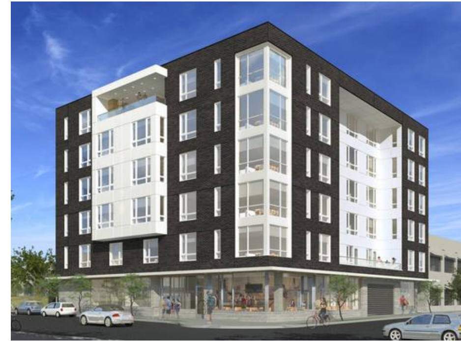
5-over-1 Example: Hoyt 20, GreenLight Development, Portland
