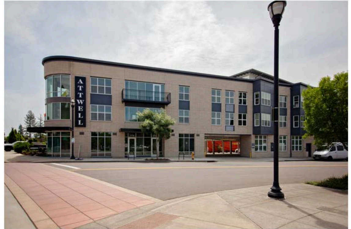
Attwell Off Main Apartments. Source: Green Light Development.
