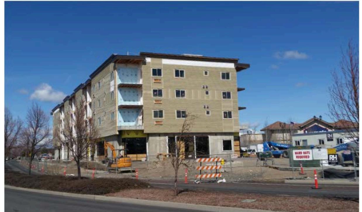
Cook Crossing in Redmond, Oregon. Source: R&H Construction
