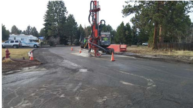
DRILLING FOR BLASTING
