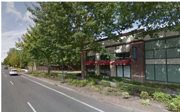
Active frontage set back from busy road
