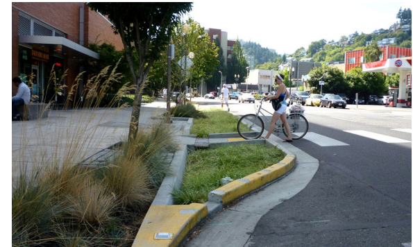
Mid-block crossing, curb extensions, stormwater treatment
