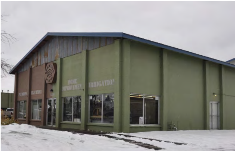
Adapted industrial shed
