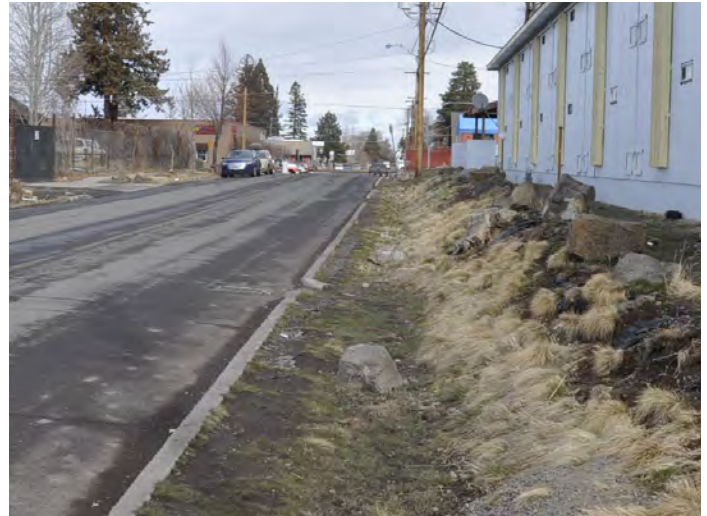
Missing sidewalks in residential and industrial areas
