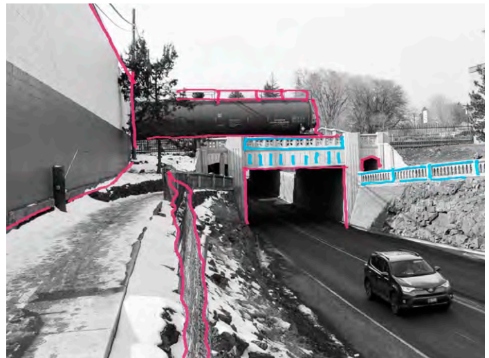
Franklin/97/RR: Narrow ped/bike route, unwelcoming edges, historic bridge details
