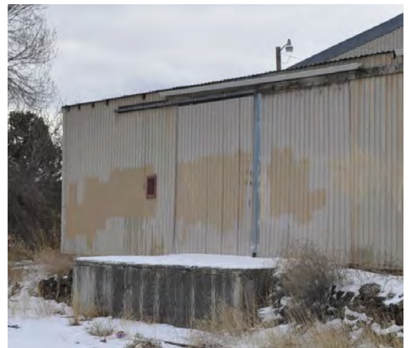
Corrugated metal sheds along railroad spur
