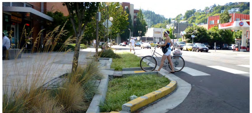
Mid-block crossing, curb extensions, stormwater treatment
