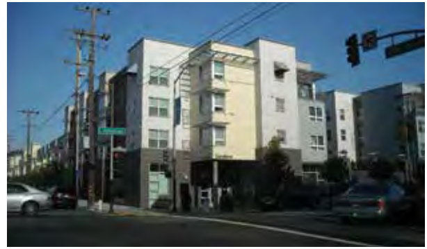
Valencia Gardens, public housing project, on 15th and Valencia Streets in the Mission, San Francisco, CA. 64 Photograph courtesy of Mark Pritchard, Flickr Creative Commons, under the following license: http://creativecommons.org/licenses/by-nc-sa/2.0/ .
