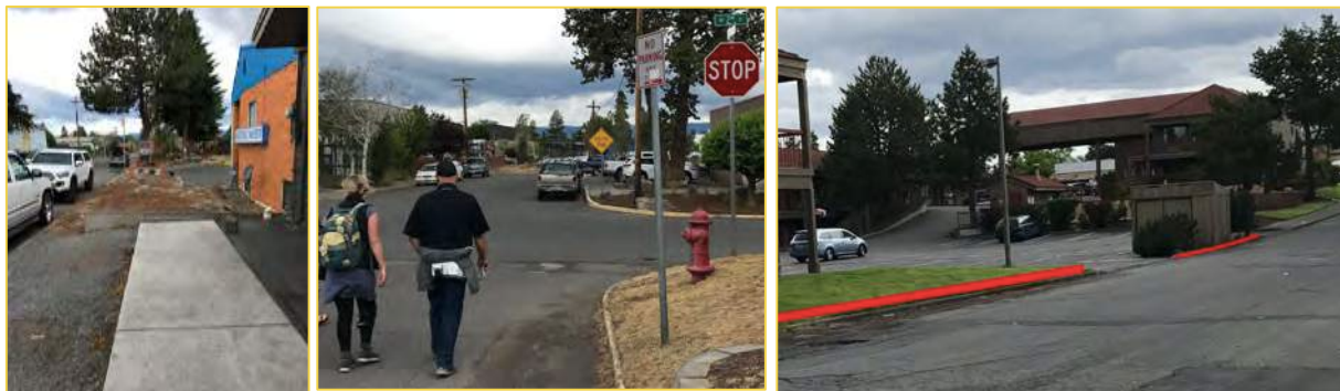
Sidewalks end abruptly or do not exist in many stretches of the BCD, forcing people to walk in the street or on private property. In the photo on the right the red line indicates where the sidewalk is missing and does not extend the length of the block.
