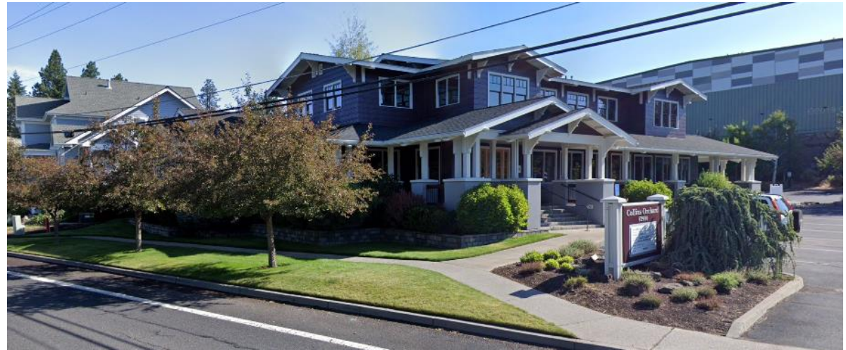
Example of marijuana testing and research facility.
