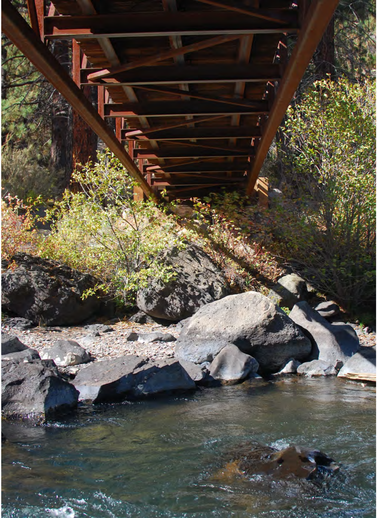
South Canyon pedestrian bridge
