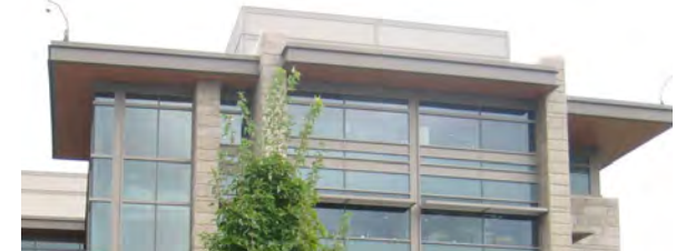
Mechanical penthouse appears to be part of the roof.
