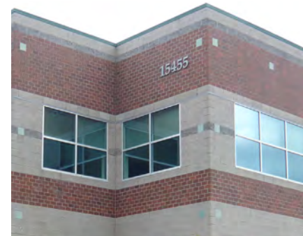
Use a combination of horizontal lines such as banding and vertical lines such as reveals to contribute to a coherent building design.
