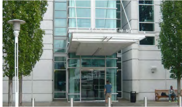
Entry is emphasized with glass, canopy, and lighting.
