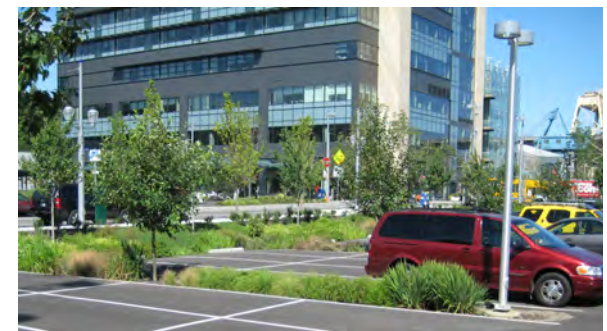
20'-tall parking lot lighting
