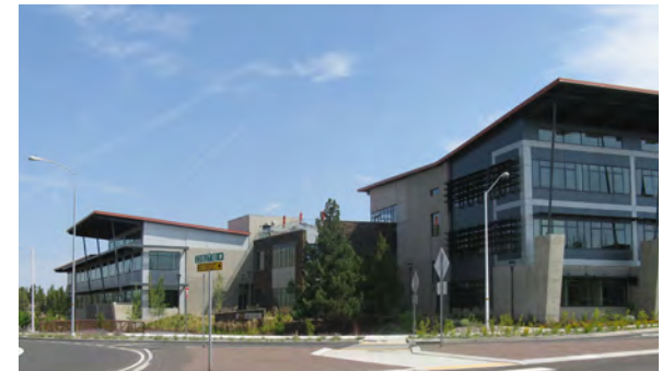
Building massing and form designed to announce entrance into a special district.
