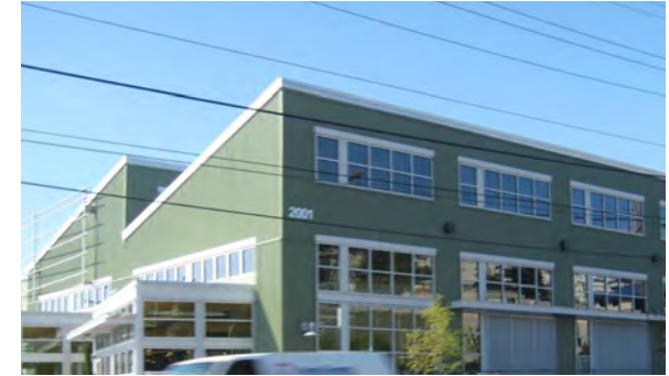
Classic industrial roof with light monitors.
