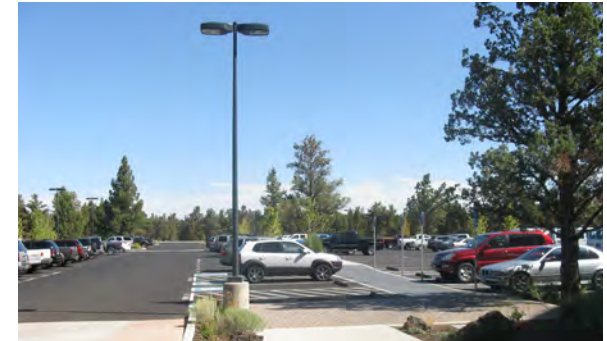
25'-tall cut-off shades, Les Schwab parking lot
