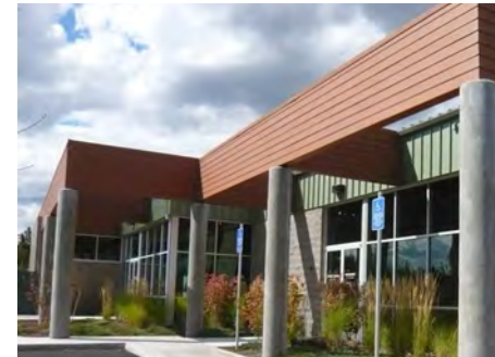
Simple columns add a layer of depth and interest to otherwise simple, flat façades.
