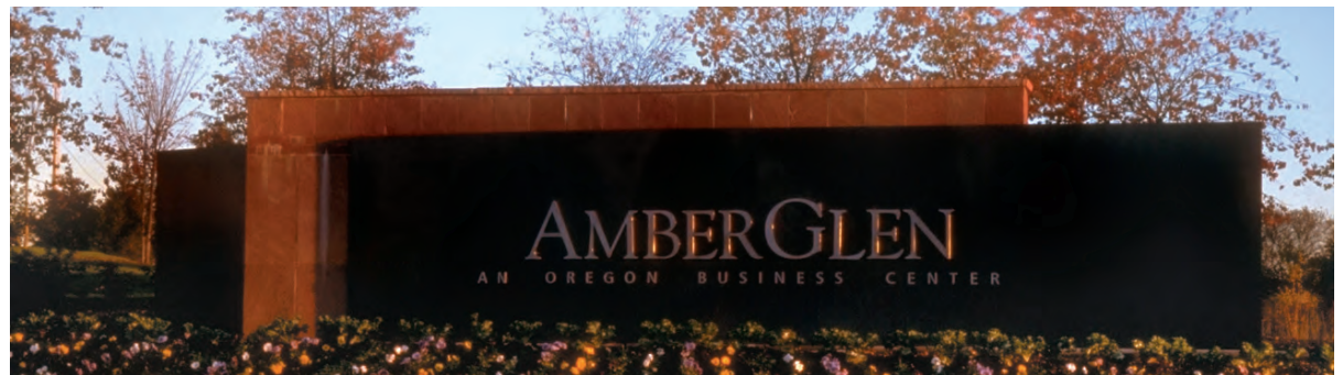
Interesting forms and contrasting textures and materials help capture attention while establishing a common vocabulary throughout the site.
