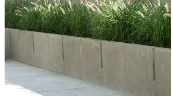
Cast-in-place concrete retaining wall with integrated planters
