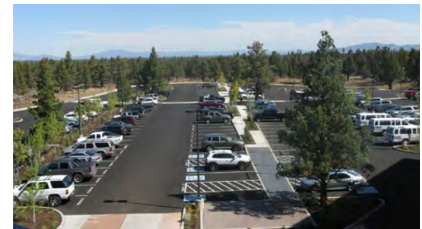
Les Schwab parking lot features pedestrian walkways, shade trees, stormwater swales and preserved native vegetation.
