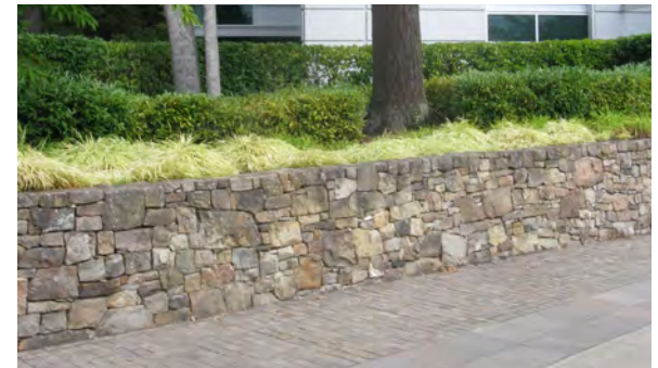
Native stone facing wall
