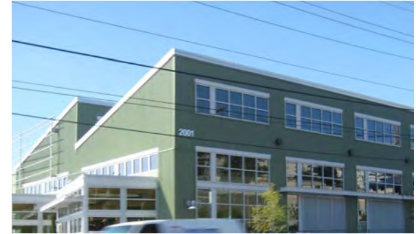
Classic industrial roof with light monitors.
