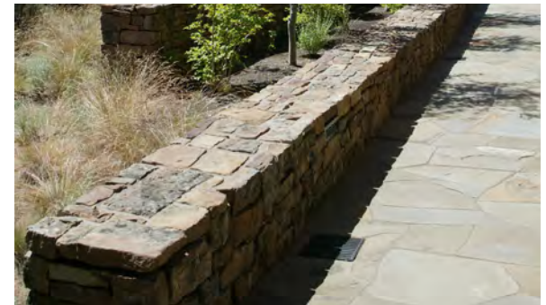
Native stone facing wall
