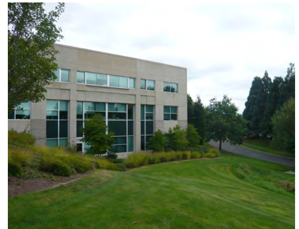
A light industrial building, fit into a sloping site.
