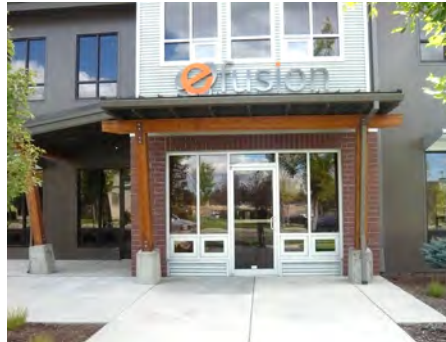
This otherwise simple building incorporates window overhangs, a portico style entry, and larger windows at the base.
