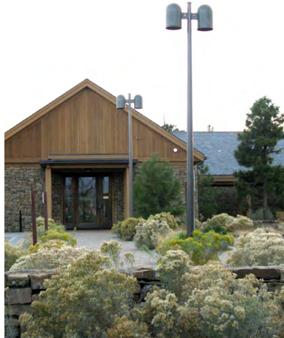
Parking lot lighting
