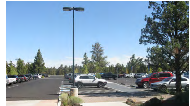
25'-tall cut-off shades, Les Schwab parking lot
