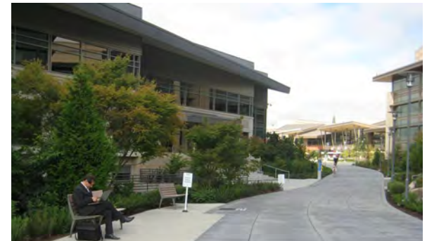
Walkways link different buildings.
