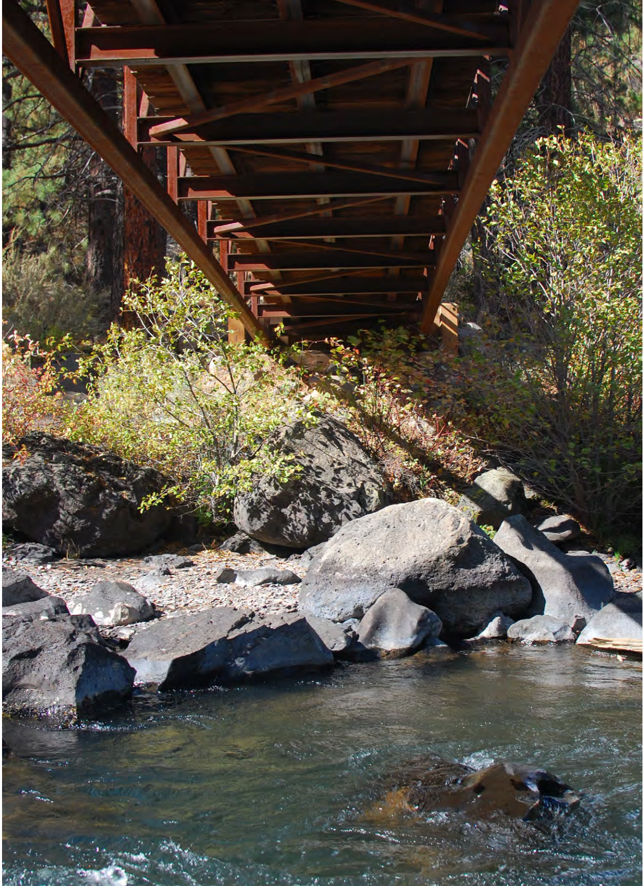
South Canyon pedestrian bridge
